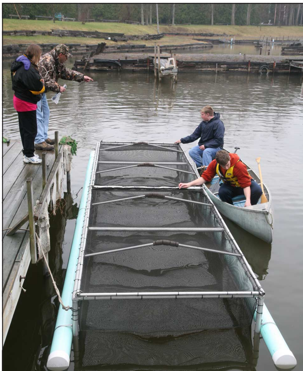
Troop 90 Scouts Ryan Moses and Arvis Collins tie down the top screen on a fish pen. The five feet wide by five feet deep by 20 feet long pens are constructed of metal piping and mesh, with poly tubes for floatation.
