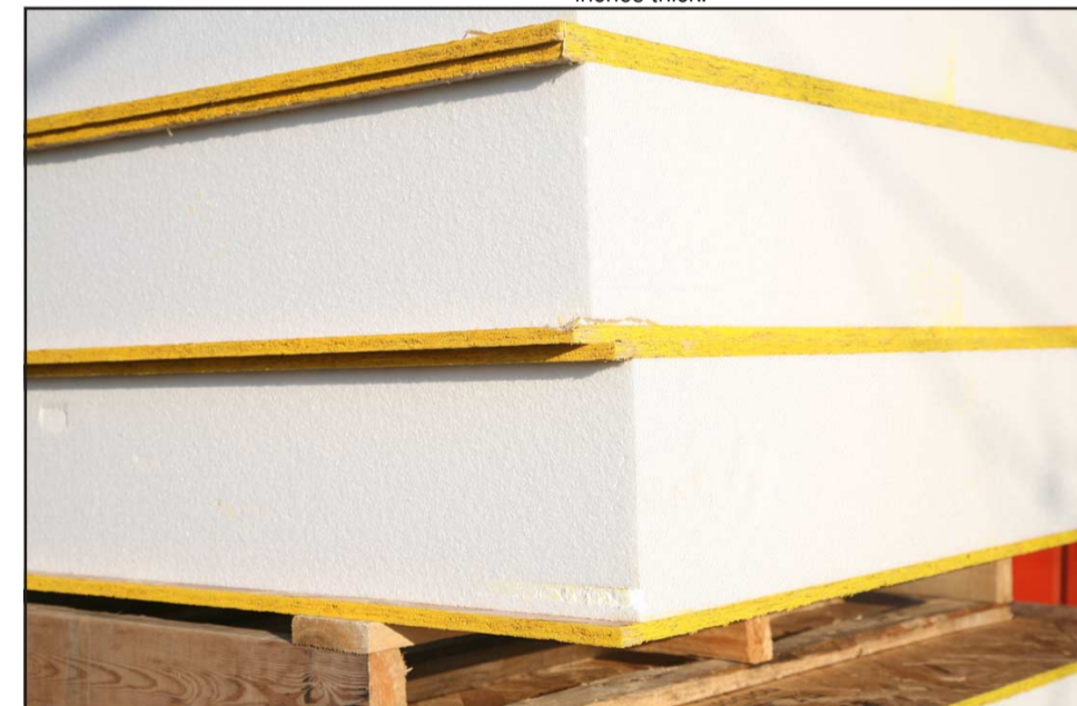
A stack of SIP's (Structural Insulated Panels) sits on a pallet. These panels will form the roof and provide an R value of about 40, eliminating the need for additional attic insulation. For this home 22 panels will be used, 11 on each side of the ridge beam. In this type of construction no trusses are used.
