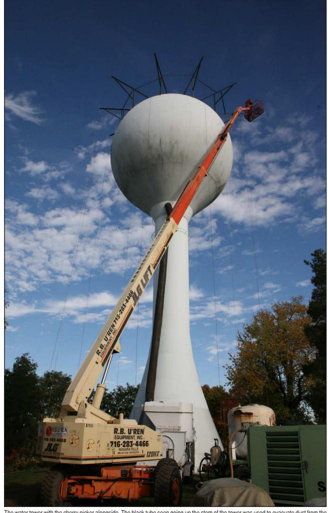
The water tower with the cherry picker alongside. The black tube seen going up the stem of the tower was used to evacuate dust from the interior while it was being sandblasted. The tank has a 250,000 gallon capacity and is now managed by Monroe County Water Authority.
