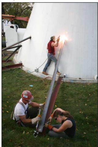
**Dan Murcin** and fellow workers temporarily attaching the base outriggers. After the job is completed the welded points will be burned off and the attachment spots will be repaired.
